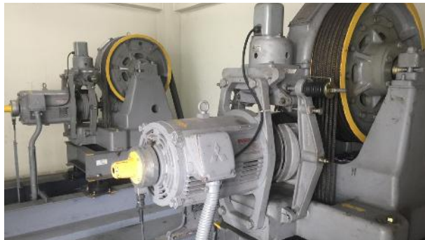
One of the accredited service providers of Mitsubishi facilitated the repair of the elevator traction machine as part of preventive assessment and maintenance.
